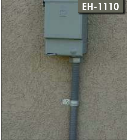
Add A/C Circuit & Disconnect
