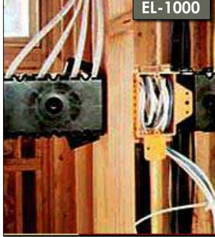
Alarm System Pre-Wire
