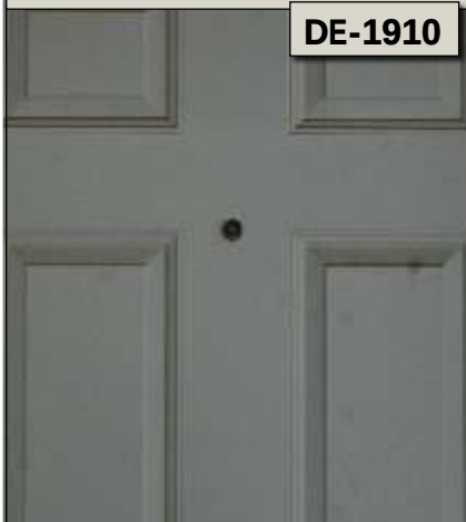
Peep Hole Installed in Entry Door
